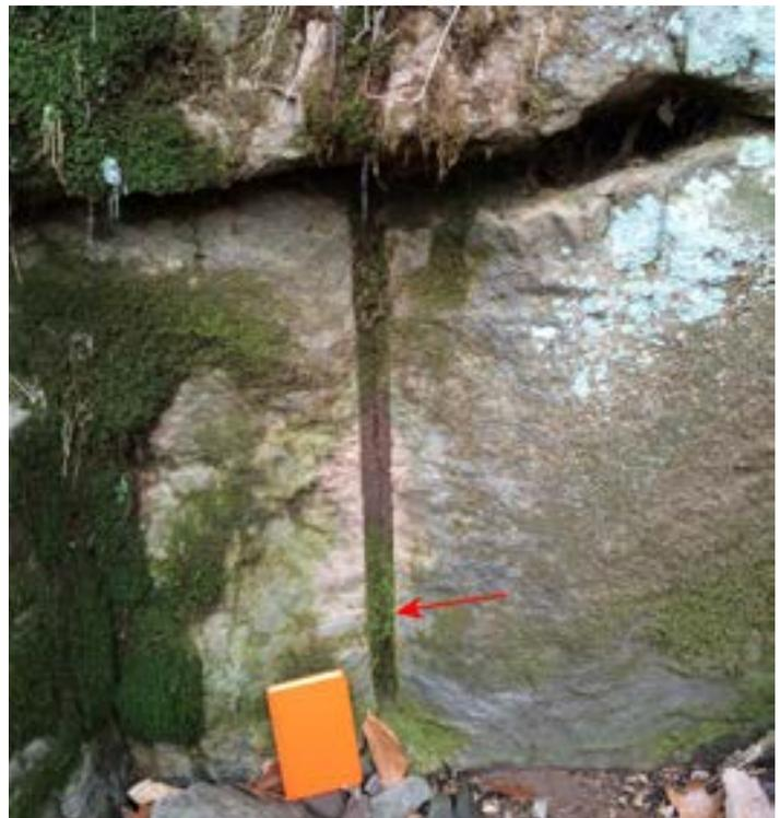
**Figure 8.** Trace of an old plug inserted into the rock face (6-inch-long field book shown for scale) at an abandoned quarry in Stockton. *Photo by F. Rea*
